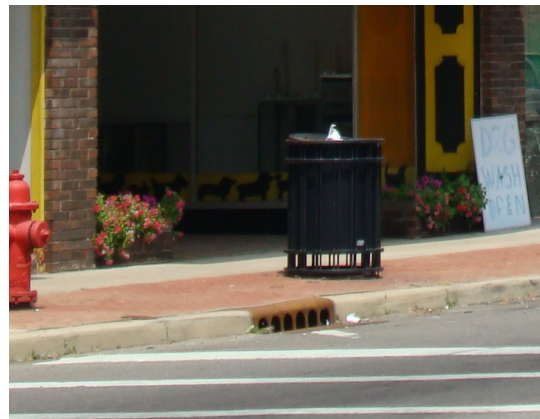
Defined gutter line and curb inlet with vertical opening that can collect surface water even if flat grate is clogged with leaves or grass clippings
