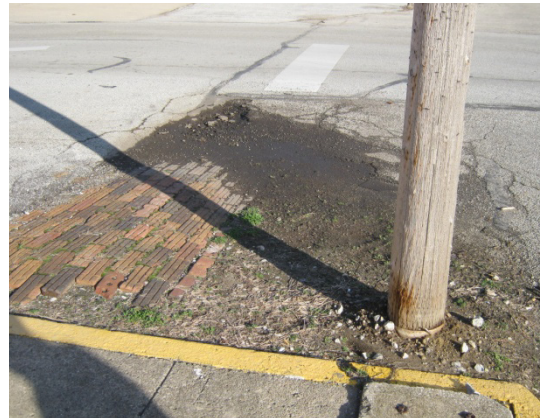
Evidence of standing water contributing to the deterioration of Indiana Street
